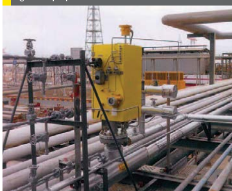
Fig 8: Sample probe cabinet site installation
