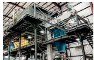
Pursell Agri-Tech's Sylacauga CRF demonstration plant.
