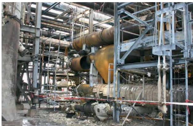
Damage caused by the explosion at the Tesoro refinery, due to HTHA corrosion.
