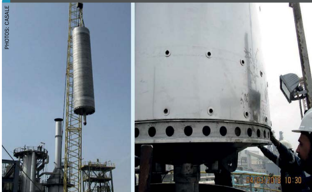
Fig. 7: Cartridge lift and installation inside converter shell
