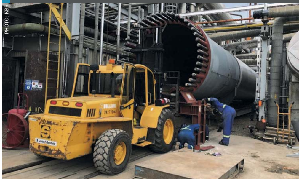
Fig. 11: Installation of new ammonia converter shell
