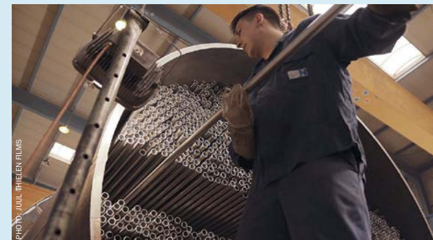
Installation of the new Safurex® Star* stripper tubes.
