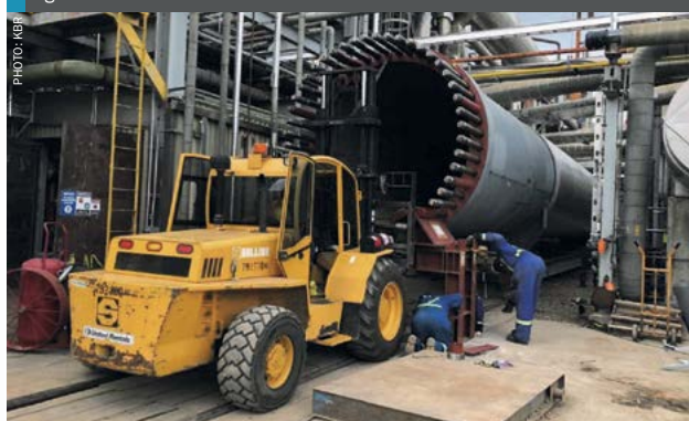
Fig. 11: Installation of new ammonia converter shell
