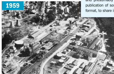
The Modderfontein ammonia complex, South Africa.
