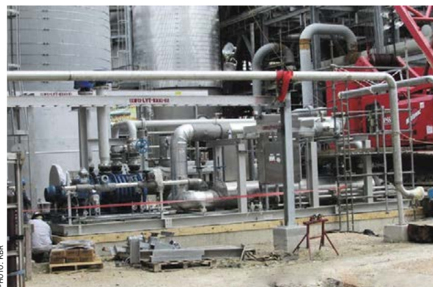
Fig. 4: Ammonia-air mixing skid during construction for a 2,300 t/d ammonia plant.
