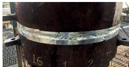
Fig. 3: Tightness test for large size flanges.
