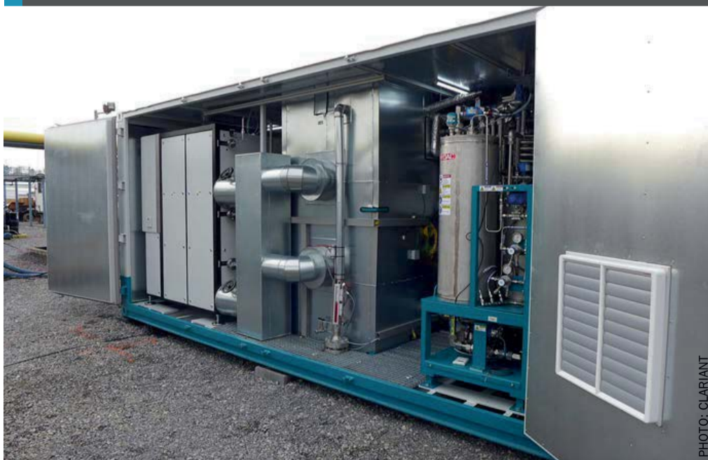
Fig. 3: LOHC installation – easy and safe hydrogen storage
