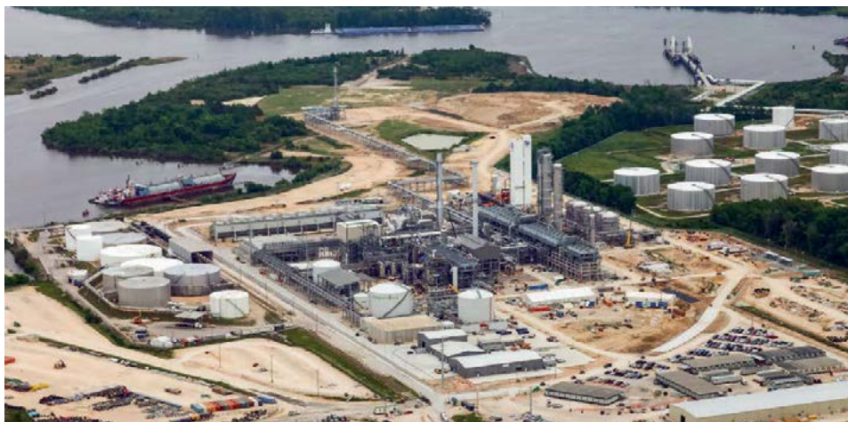
The Natgasoline methanol plant at Beaumont, Texas.
