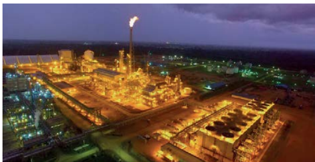
Another view of the Indorama facility.
