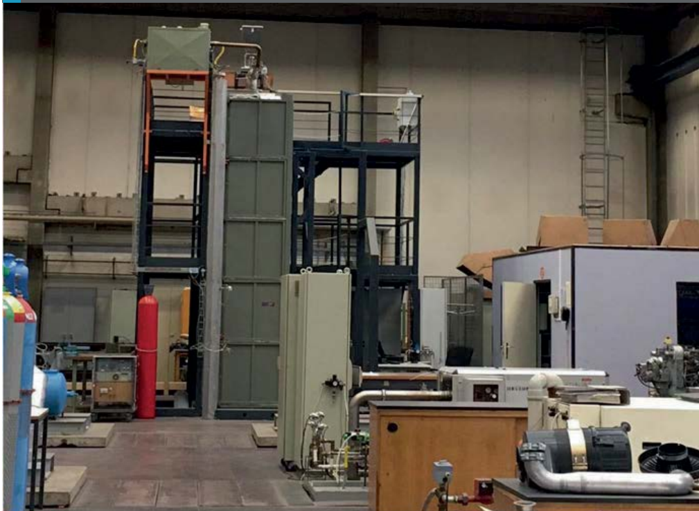
Fig. 5: Pilot plant under installation
