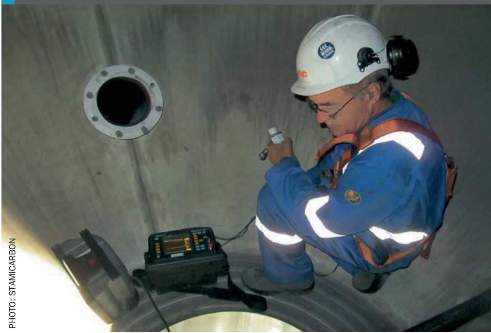
Fig. 5: Plant and equipment inspections are vital
