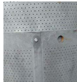
Fig. 15: Two sections of the central distributor joined together
