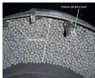
Fig. 21: Annular layer of inert balls between distributor and catalyst
