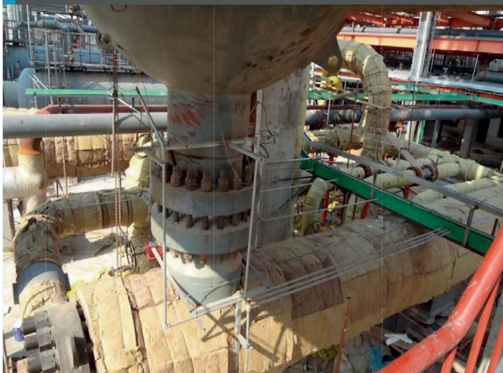
Fig. 4: Direct connection with BFW preheater
