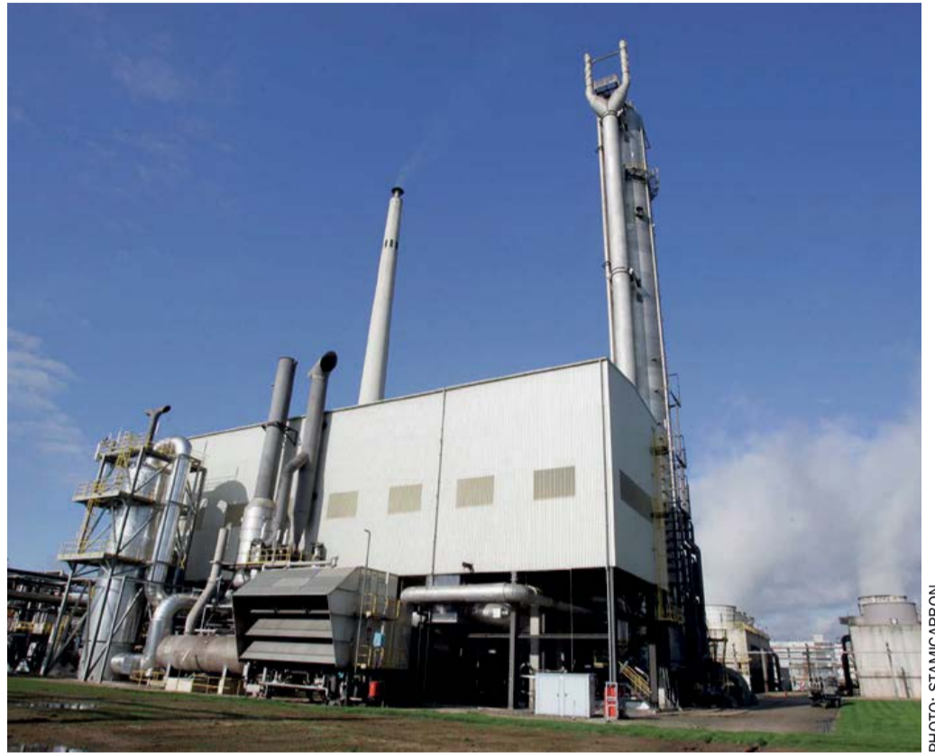
Fig. 4: Dual pressure nitric acid technology plant in operation since 1989.
