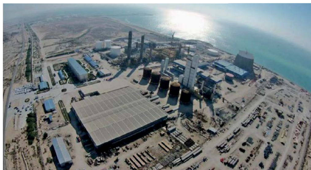
Fig. 1: Construction of world's largest methanol plant, 7,000 t/d with Casale technology.
