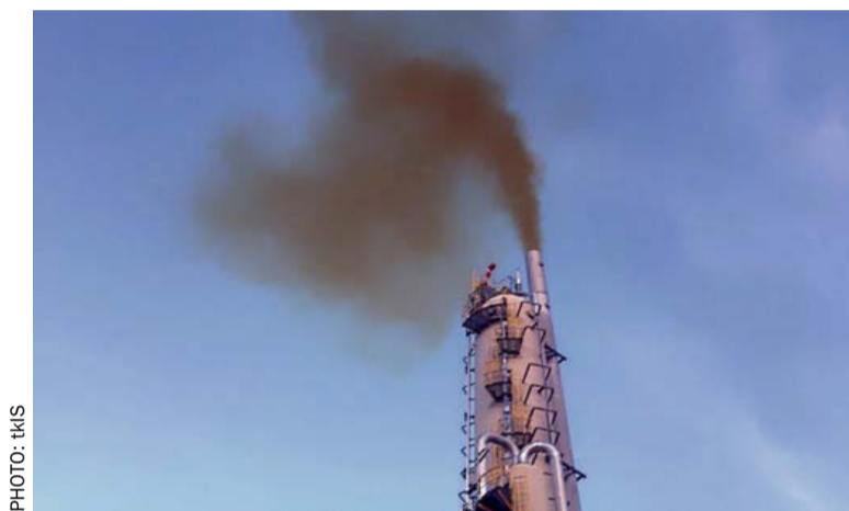
Fig. 3: Brownish plumes during start-up.
