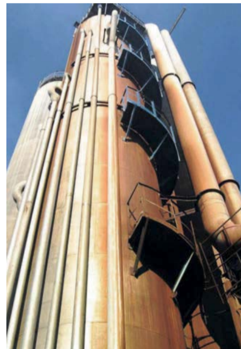
Fig. 1: Nitric acid plant Azomures Line II: Oxidation towers (2 brownish coloured columns at the front) for cooling and oxidation of NO to NO 2 ; and absorption columns (2 columns at the back, of which just one is visible) for absorption of NO x .
