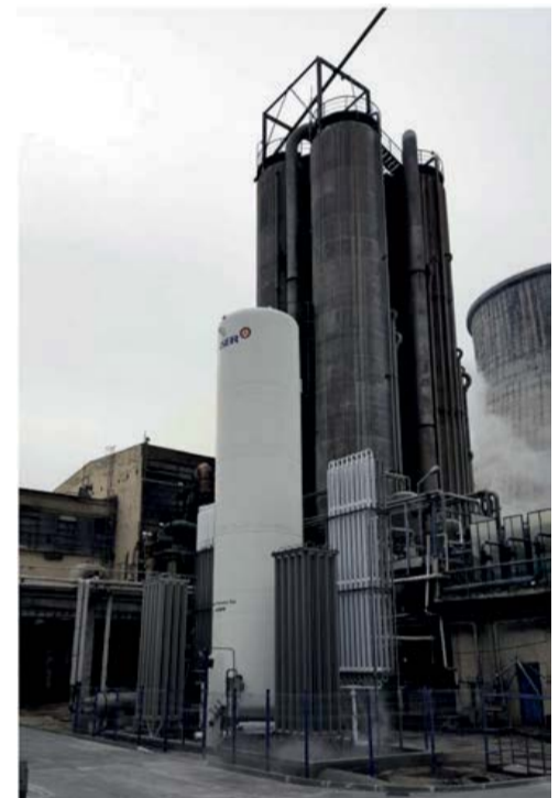
Fig. 7: Nitric acid Line II at Azomures site with the final installation of Oxyboost Technology.
