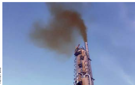
Fig. 3: Brownish plumes during start-up.
