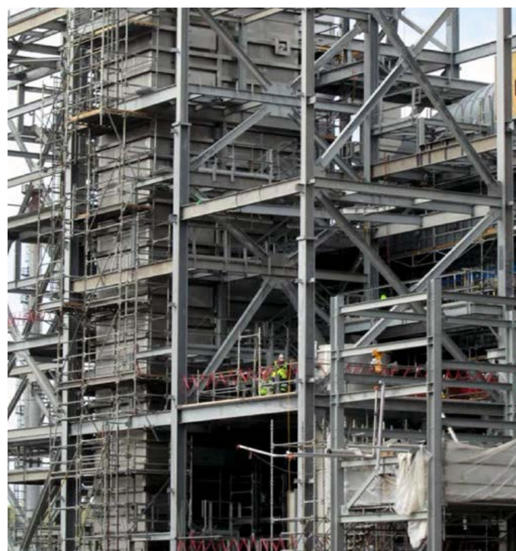
Fig. 8: Construction phase of a rectangular modularized MMV scrubber installation for a 1,000 t/d urea granulator.
