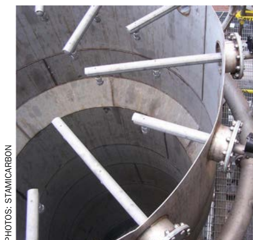
Fig. 3: View of a typical SpiralMist quench stage.
