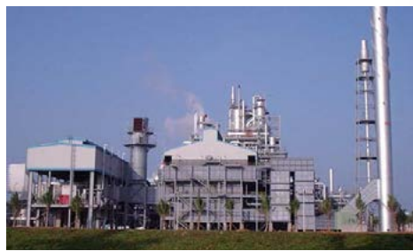
Fig 8: KBR Purifier gas turbine integration scheme at CNOCC, Dongfang, Hainan Province, P.R. China (began operation in 2003).
