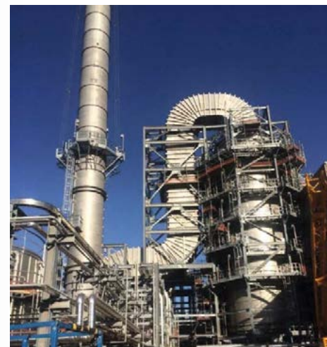
Fig. 7: Construction phase of a MMV scrubber/WESP installation for a urea granulator.
