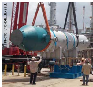
Installing a distillation tower at LyondellBasell's Channelview methanol plant.
