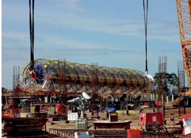
Construction of the SAMUR urea plant, Malaysia.
