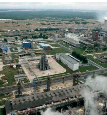
Grupa Azoty's nitrogen facility at Pulawy.
