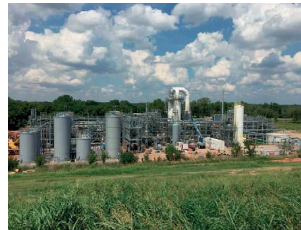
The ENVIA GTL plant at Oklahoma City.
