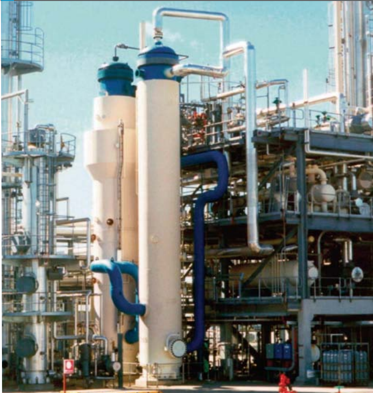
Fig 4: Gas heated reformer (GHR) and secondary reformer at Coogee, Australia
