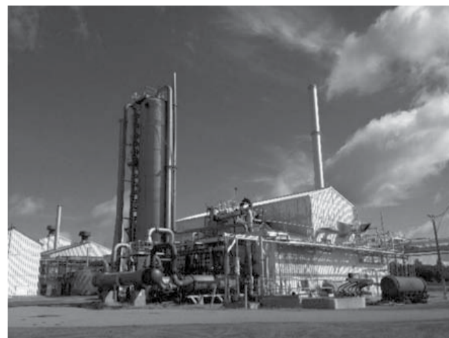
500 TPD Nitric Acid Plant, Weatherly
