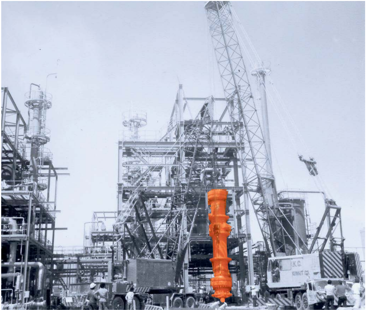
Late seventies, Kuwait Melamine plant under construction
