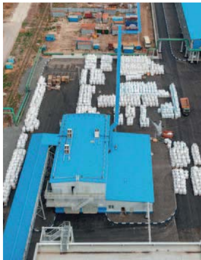
Cover: Urea bagging plant in Russia. saoirse2013 / shutterstock.com
