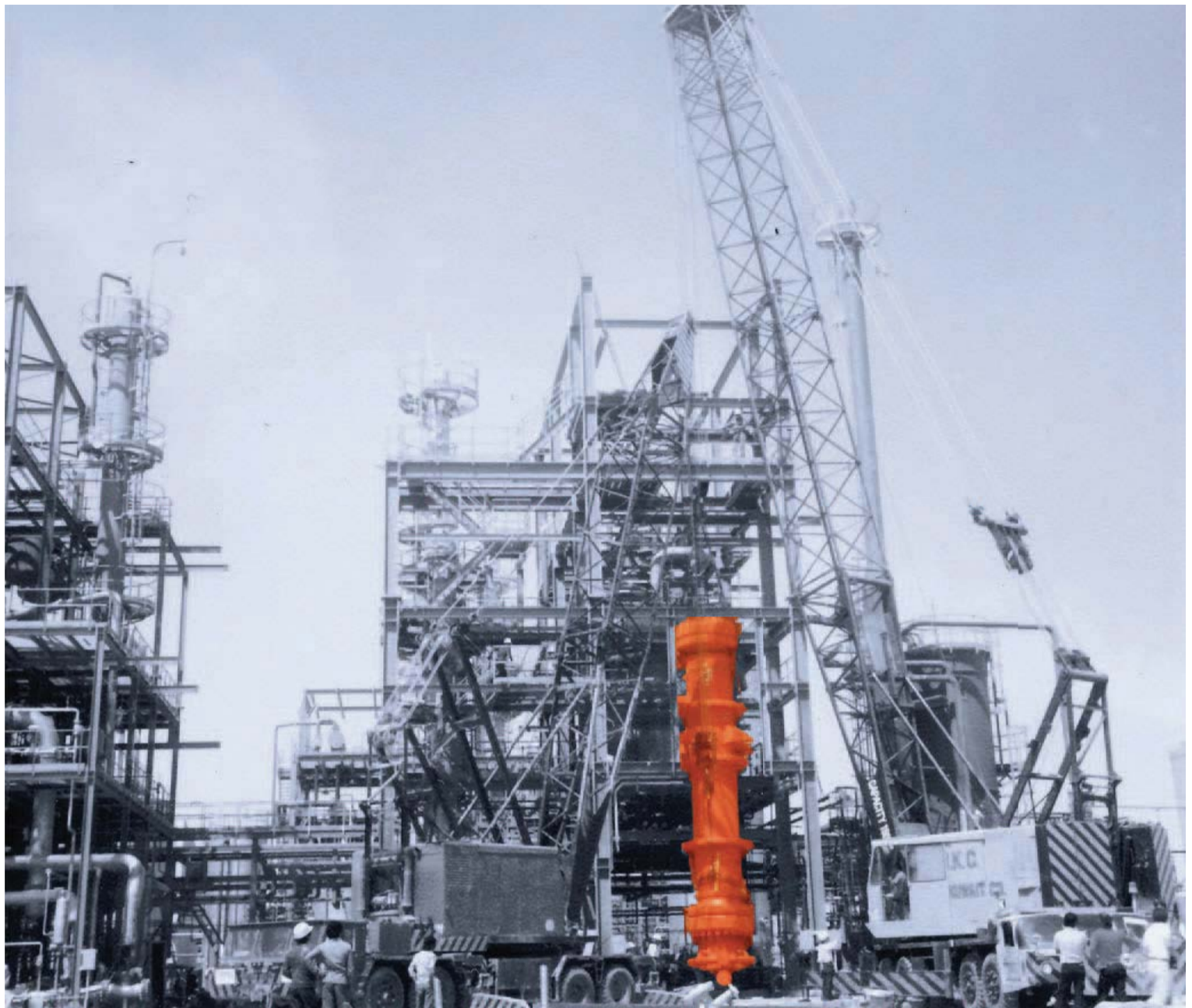
Late seventies, Kuwait Melamine plant under construction
