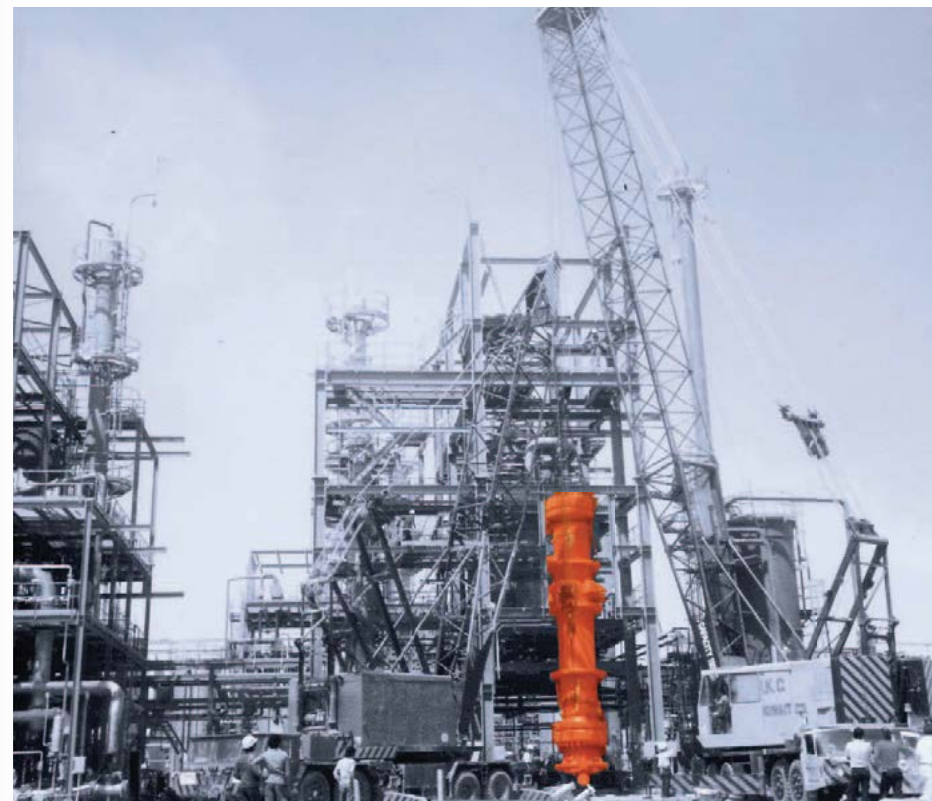
Late seventies, Kuwait. Melamine plant under construction
