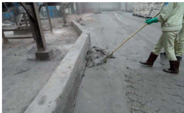
Fig. 11: Results of spills and high traffic in a fertilizer plant in the tropics.
