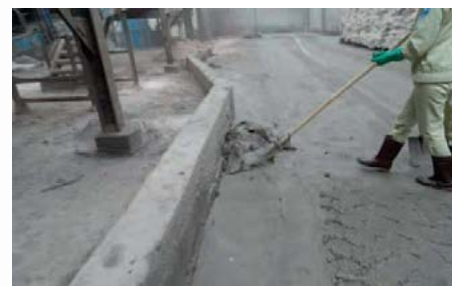
Fig. 11: Results of spills and high traffic in a fertilizer plant in the tropics.
