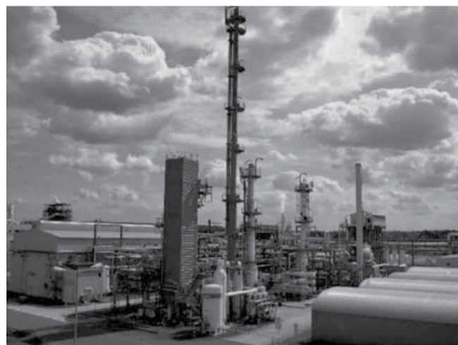
13,200 Nm³/hr Hydrogen Plant
