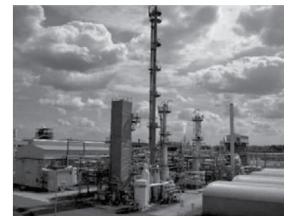
13,200 Nm³/hr Hydrogen Plant
