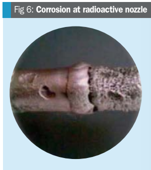
Fig 6: Corrosion at radioactive nozzle
