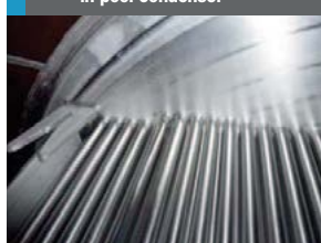
Fig 9: Excellent condition of tubes in pool condenser
