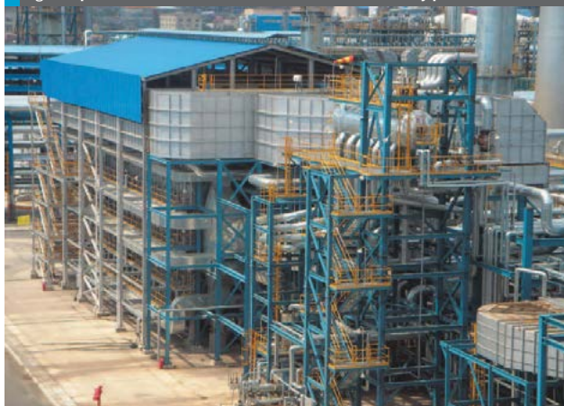
Fig 1: Topsoe side-fired steam reformer – waste heat recovery placed at side
