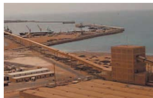
The Lifeco plant at Marsa El Brega.
