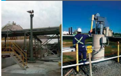
Fig 7: Periphery detection at ammonia storage area (left) and plant boundary (right)
