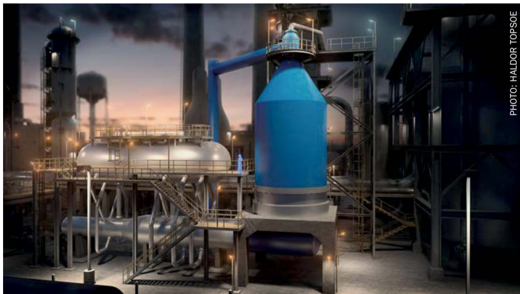
Topsoe’s SynCOR Ammonia™ technology is capable of reducing steam throughput by 80 percent.
