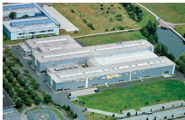
Köppern's manufacturing plant in Hattingen, Germany.
