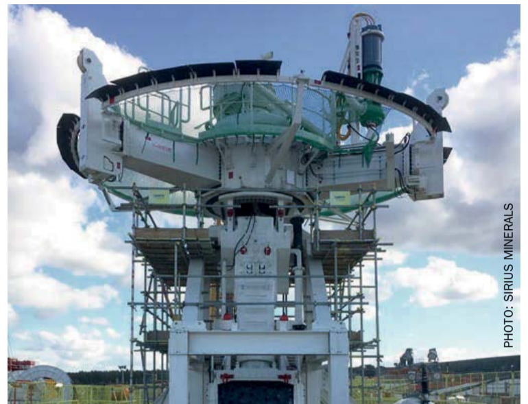
Vertical shaft sinking machine (VSM).
