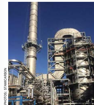
Fig. 6: Construction phase of a MMV scrubber/WESP installation for a urea granulator.
