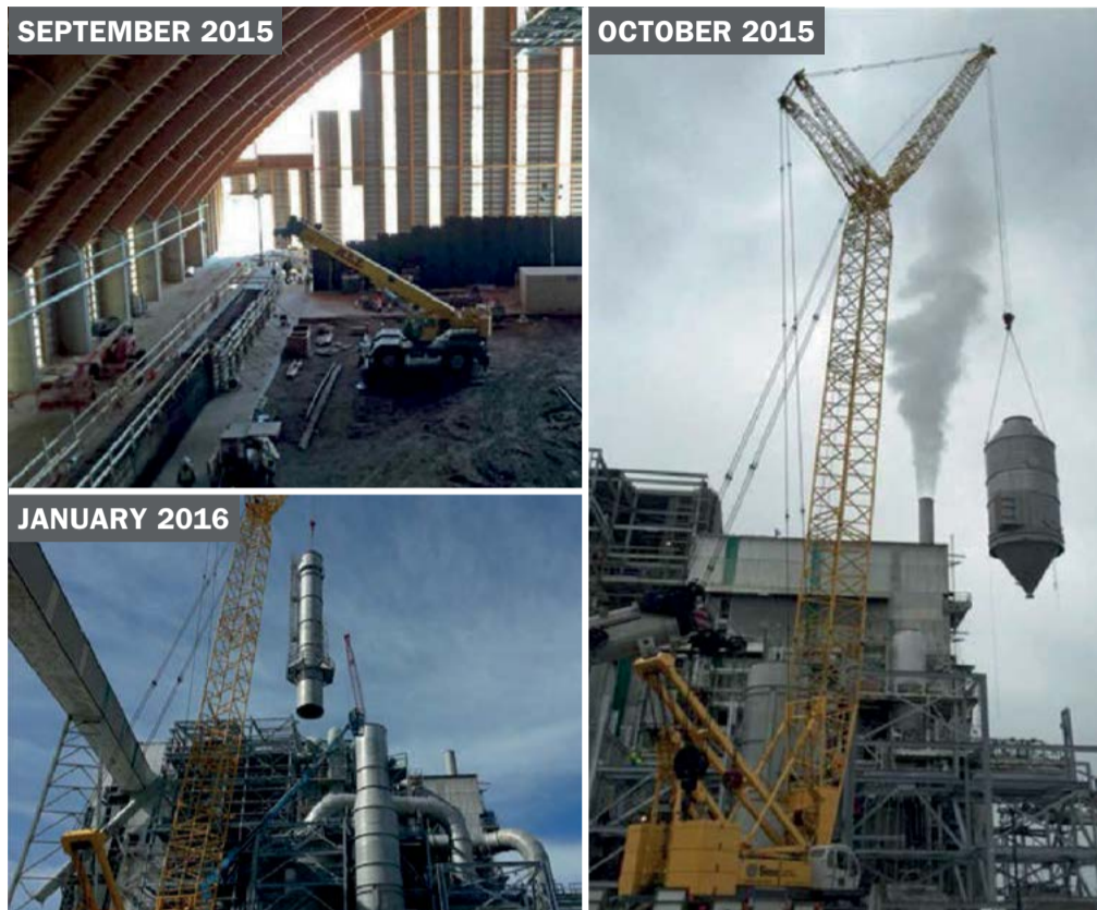
Clockwise from top left: warehouse finishing, installing scrubbers, new stacks.
