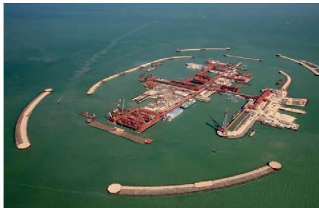
One of the artificial island platforms, Kashagan.
