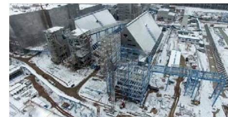
Ore and finished product storage buildings, Usolskiy.
