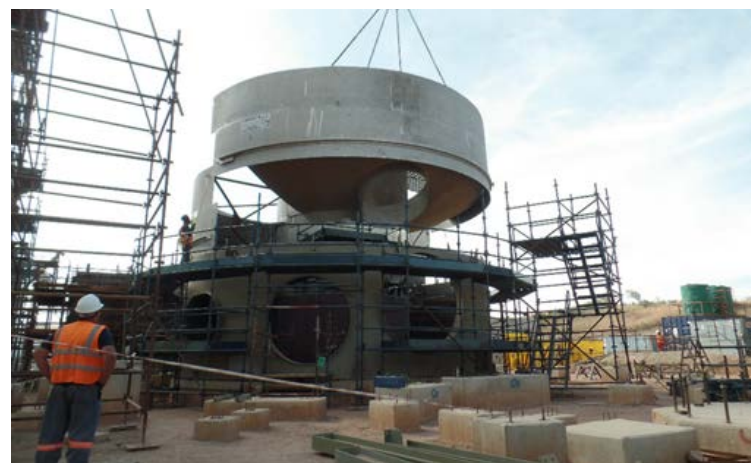
Fig. 5: Converter modules assembly in-field.
