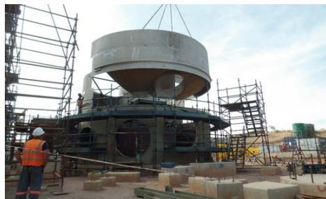
Fig. 5: Converter modules assembly in-field.
