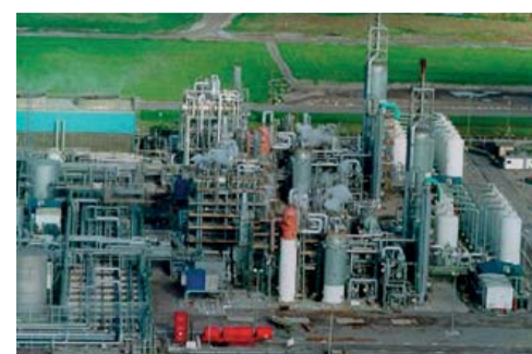
Fig. 1: The two LCA plants at Sevenside (shutdown 2008).
