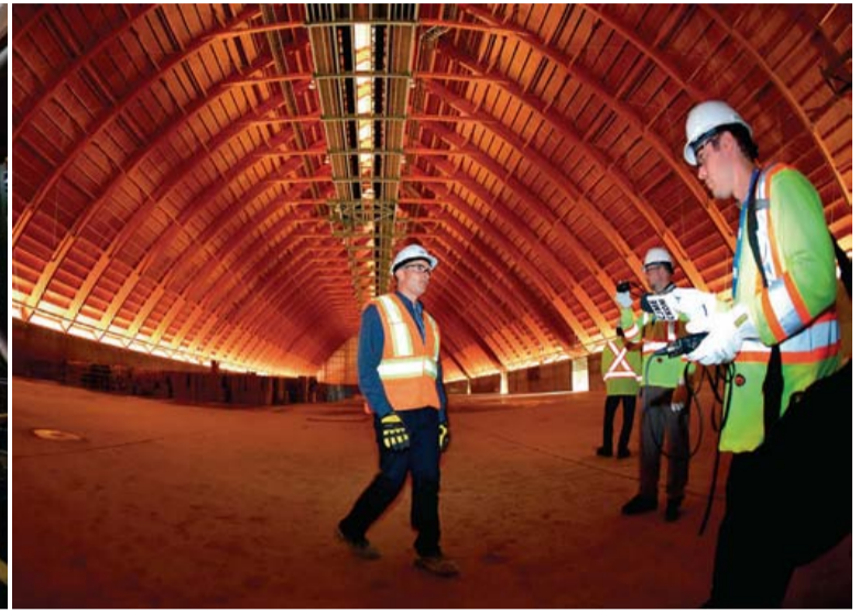
Inside the huge potash warehouse at the site.
