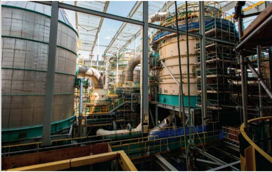
Processing plant steel work and equipment.
