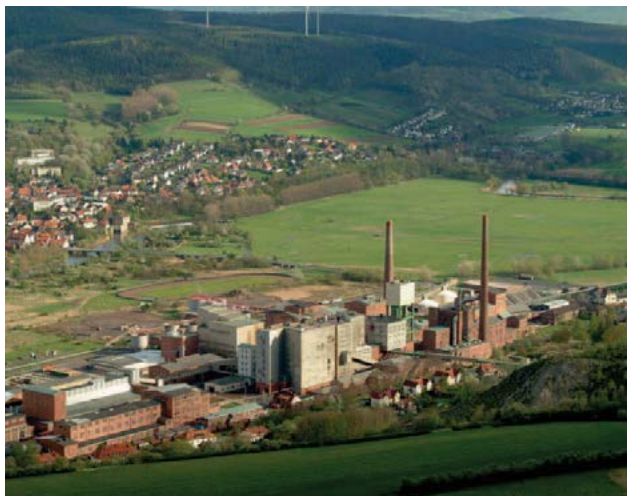
K+S Kali's Wintershall plant.
