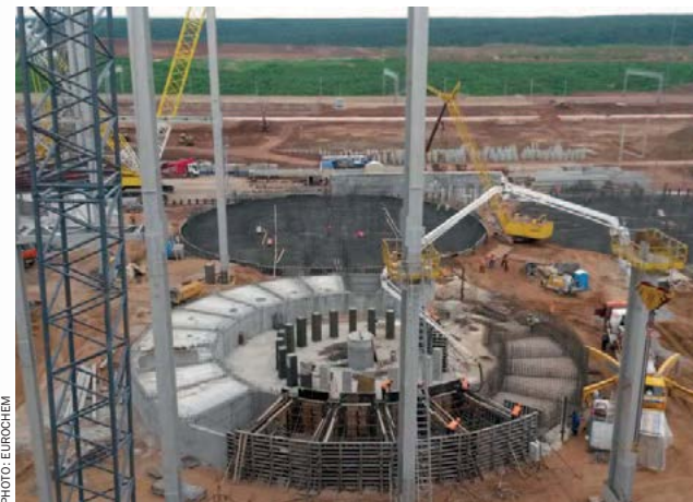
Construction at EuroChem's Usolskiy project.
