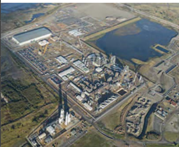
Aerial view of the Air Products' renewable energy facility.
