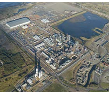
Aerial view of the Air Products' renewable energy facility.
