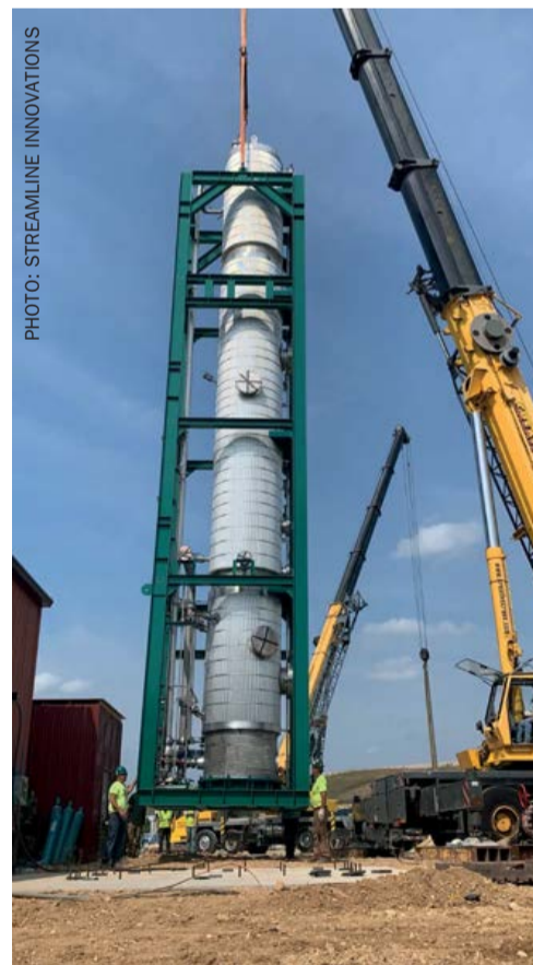
Packed tower installation.
