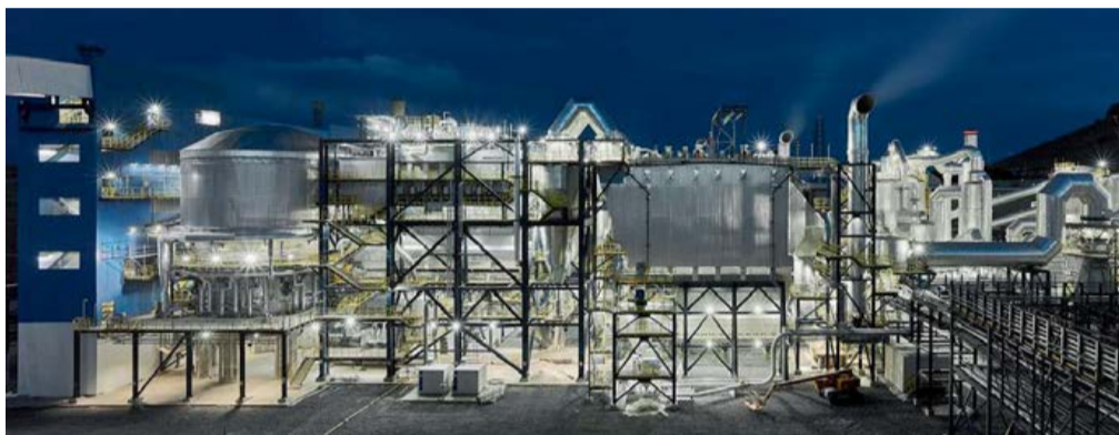
Mazidagi's roasting-gas cleaning-acid plant sections.
