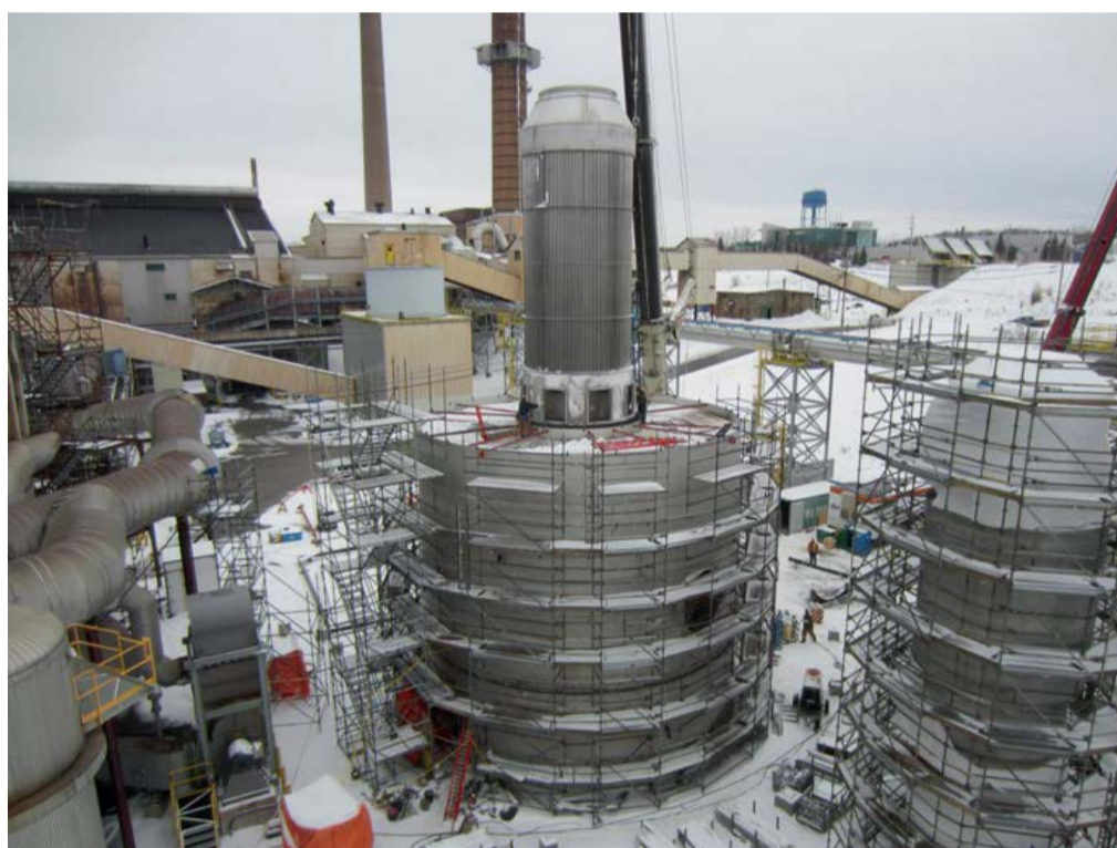
Fig. 4: Chemetics stainless steel converter with internal exchanger.
