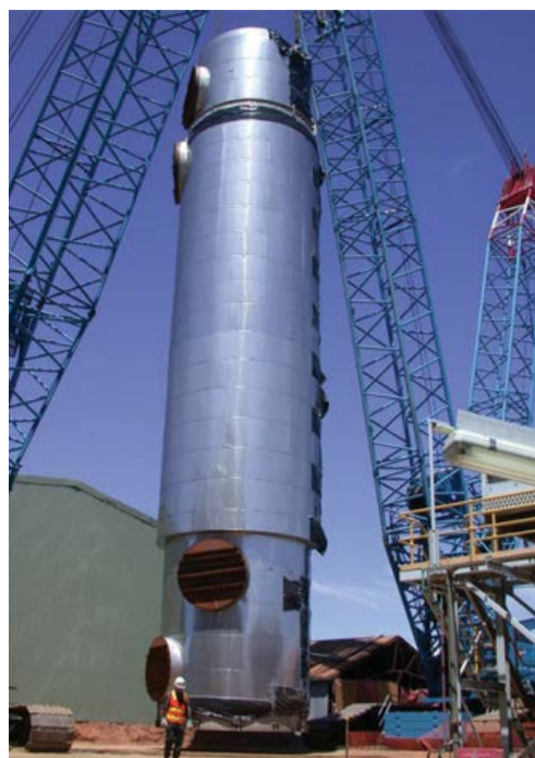
Fig. 2: Radial flow gas exchangers.
