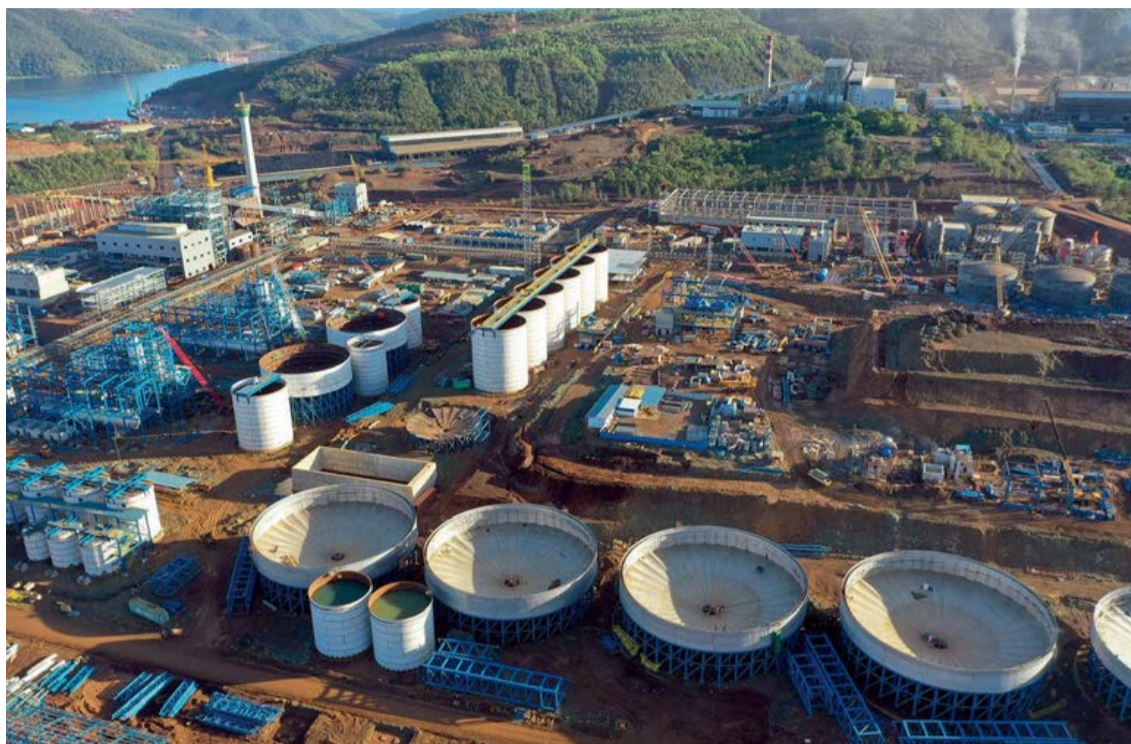
Right: The Obi Island HPA plant under construction.
