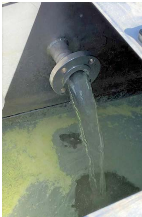
Above: Fig. 4: SG20 drum (left). Fig. 5: Scrubber waste discharge to seed generation system (centre). Fig. 6: Exhaust stack (right).
