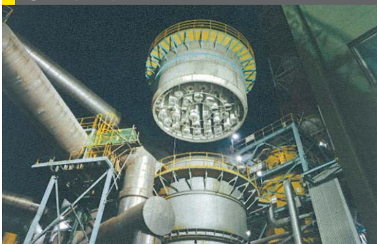
Fig. 1: Top compartment retrofit
