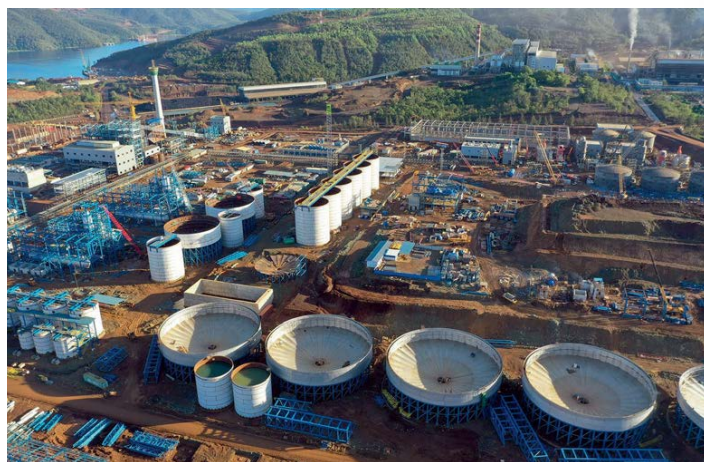
Right: The Obi Island HPAL plant under construction.
