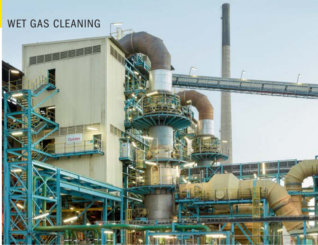
Fig. 2: Metso Outotec's Otovent venturi scrubber
