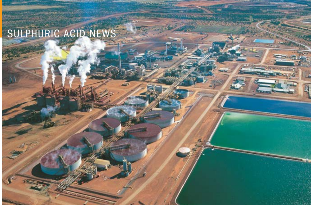
The Murrin Murrin HPAL facility.
