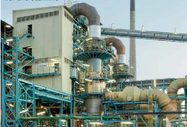
Fig. 2: Metso Outotec's Otovent venturi scrubber
