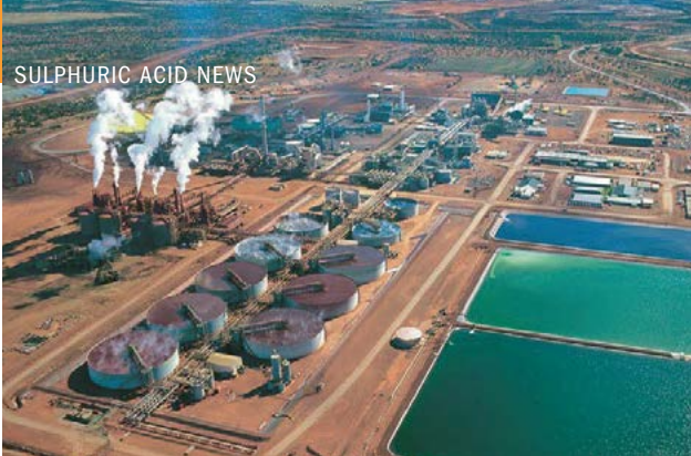
The Murrin Murrin HPAL facility.
